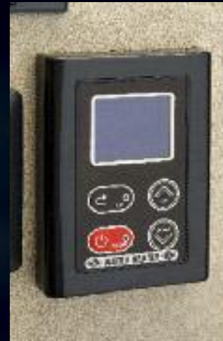
Tankless water heater control
